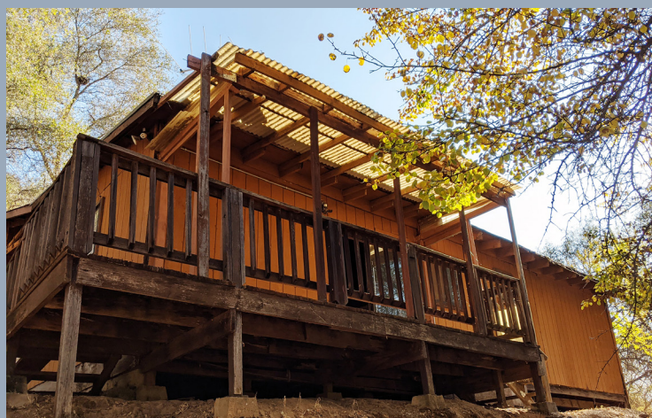
The duplex remodel project has been fully funded.
